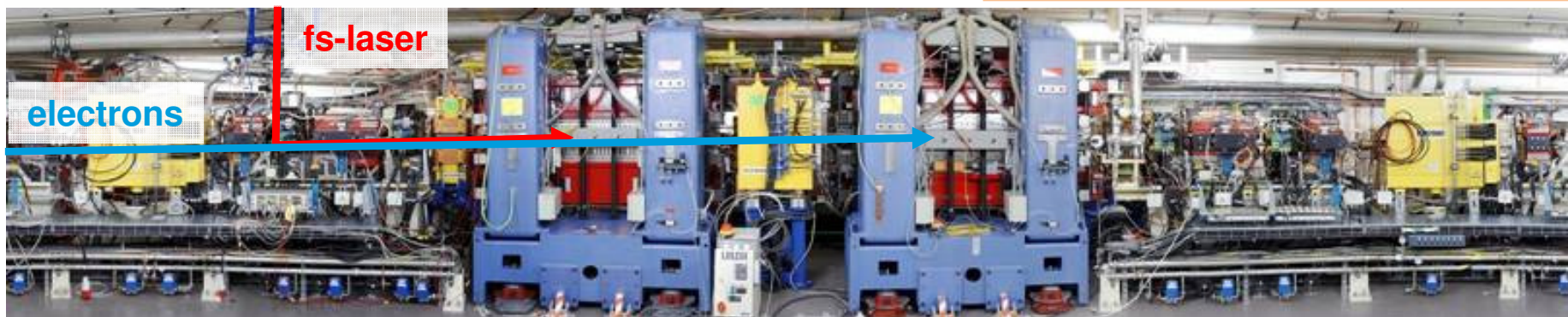
Slicing facilities in the storage ring
